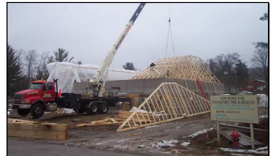
Building Under Construction
